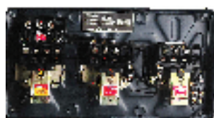
Interior View of MK1 FASD
