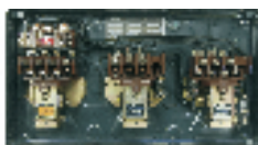
Interior View of MK2 FASD
