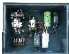
Interior View of MR-G2W
